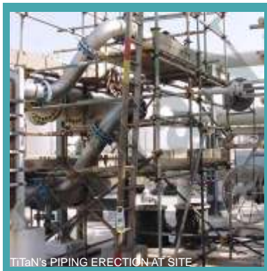
TiTaN's PIPING ERECTION AT SITE
